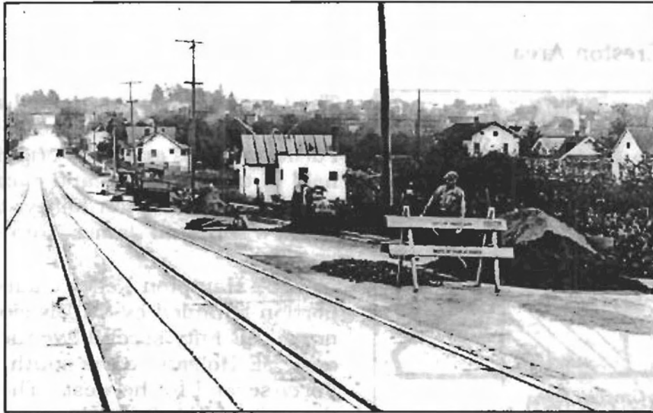
A 1931 photo showing sewer repairs at SE 35th and Gladstone, and the trolley tracks
