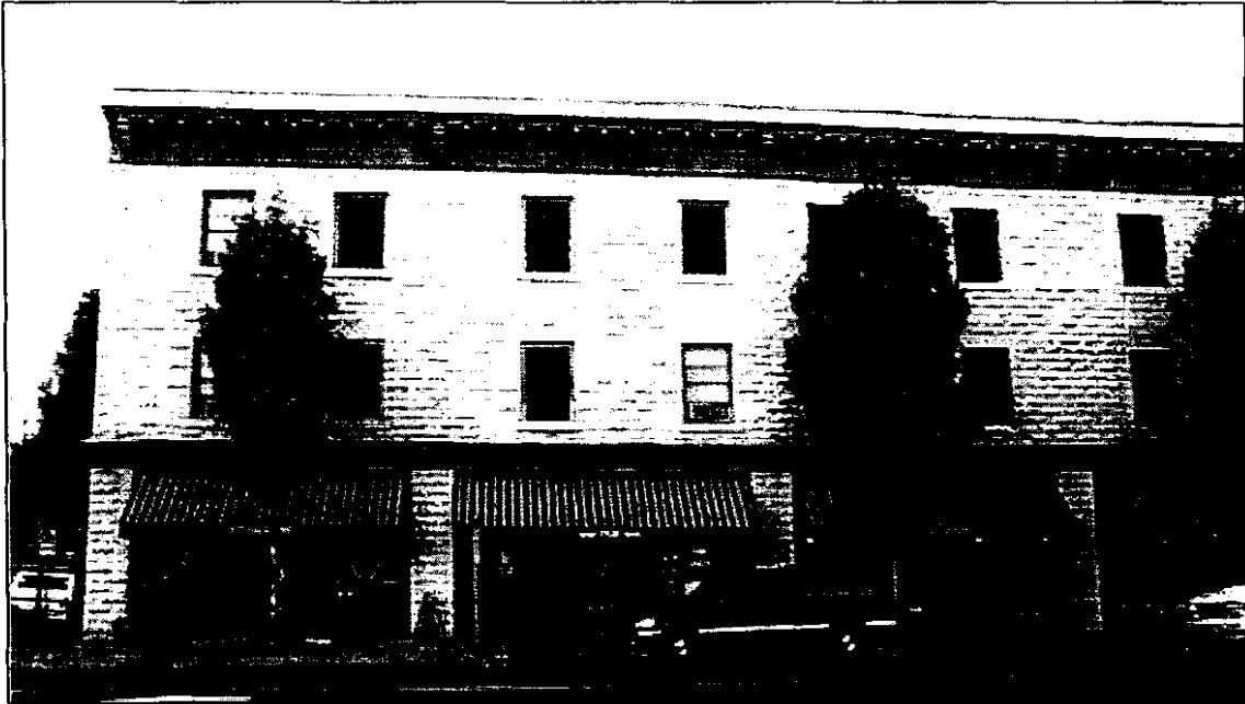
The Kenton Hotel was one of the first buildings to be renovated along Denver Avenue.
