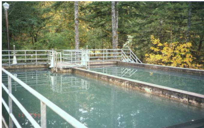
View of inlet end of settling tanks
