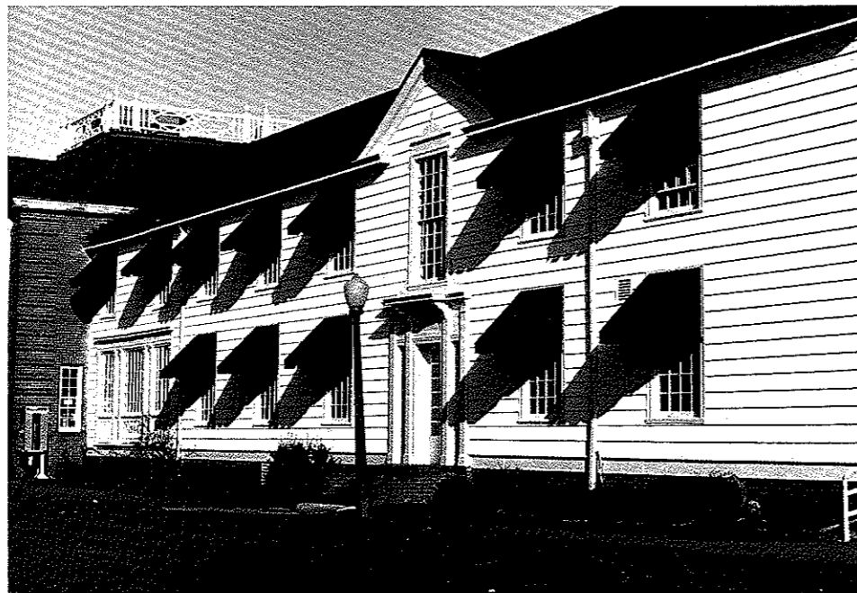
The Sharper Image: the old west wing of the music school sports a new roof, new siding, new awnings, and a fresh coat of paint. Photo by Scott Barkhurst.
