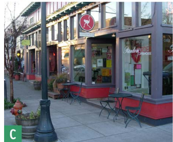
A – Building entrance oriented to the corner B – Art as a gateway element C – Improved storefront
