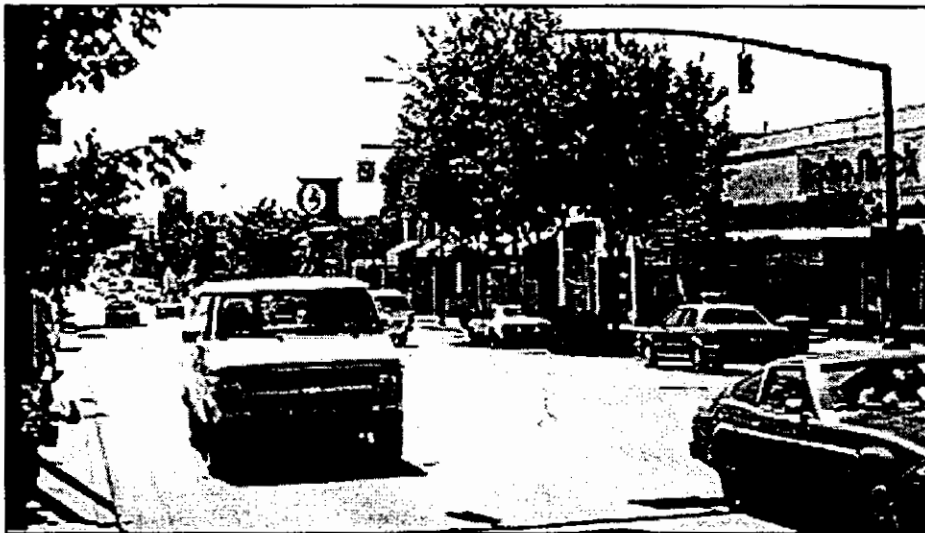
Development along the Sandy Boulevard main street is auto-oriented.
