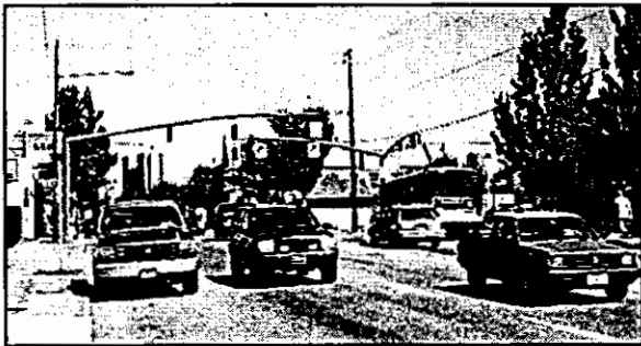
While other parts of Northeast Broadway Street have received pedestrian amenities, the street is primarily auto-oriented in the EPCP area.
