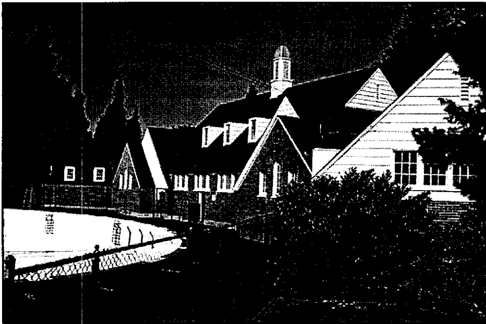
The Sellwood pool and poolhouse, designed by Ellis Lawrence, built between 1910 and 1914.
