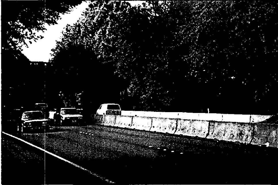
McLoughlin Boulevard at the Bybee overpass, looking south.
