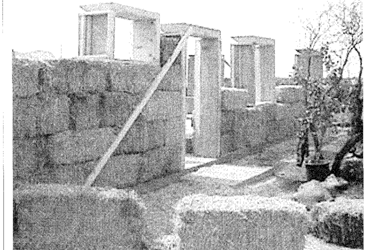
Initial framing gets under way for the Campbell home
