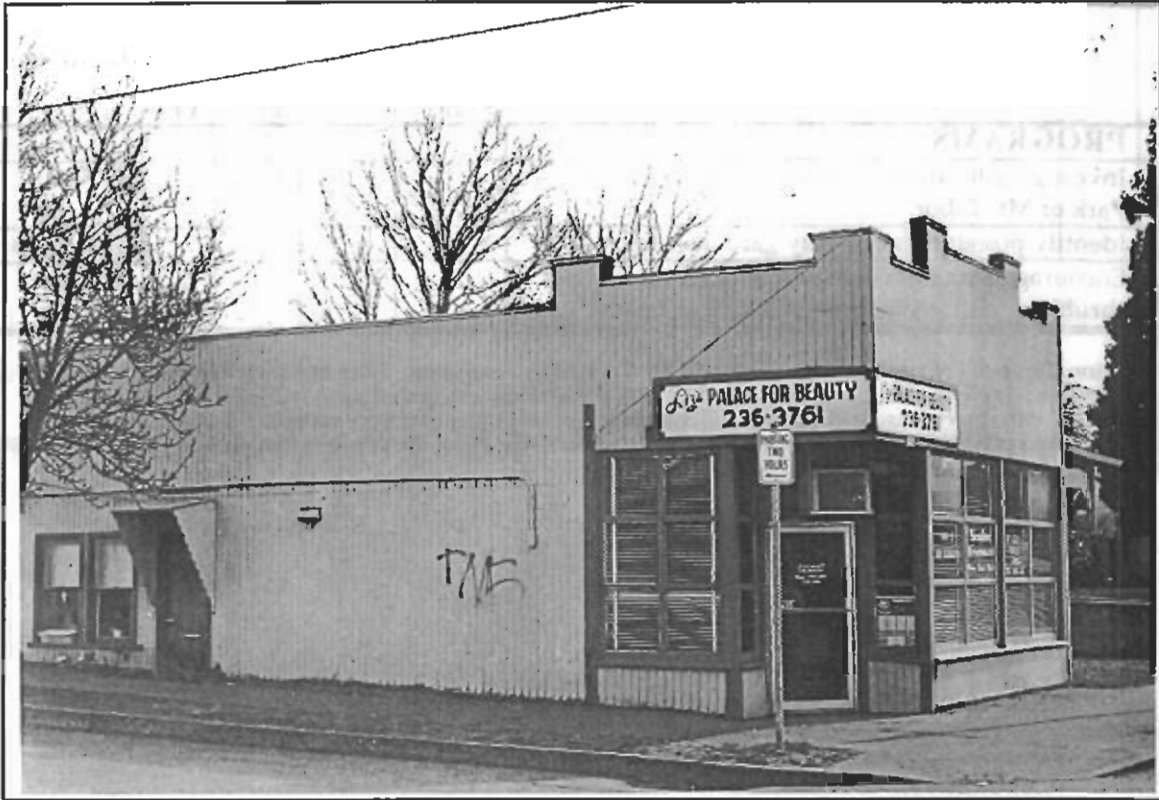
This storefront on 52nd Avenue is an example of Streetcar Era Commercial style.
