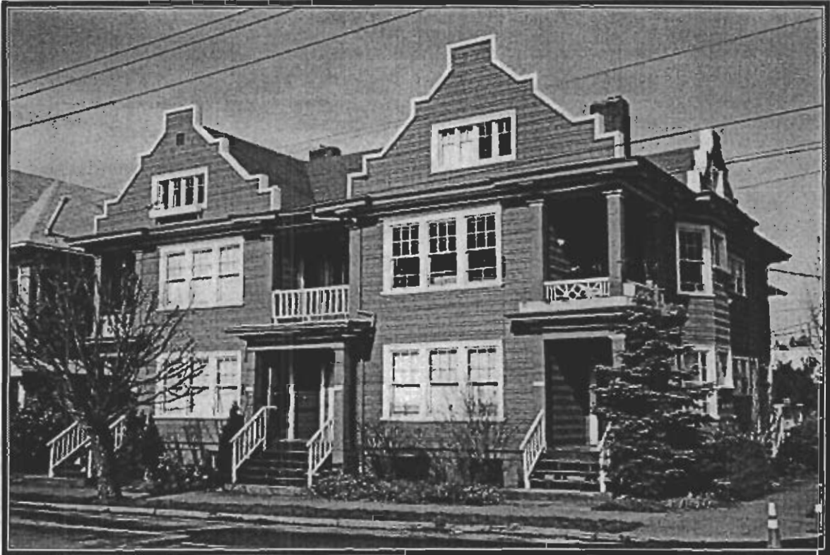
Example of renovated multifamily home in Sunnyside
