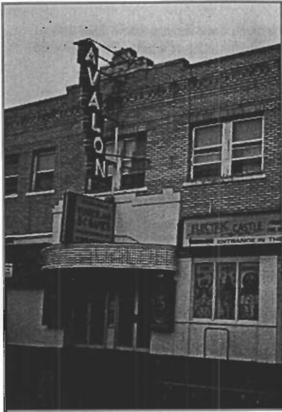
Right: Example of a Streetcar Era commercial structure, built in 1912.
