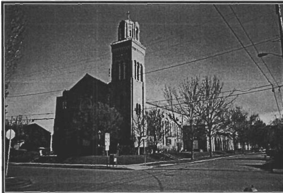
St. Stephen's Catholic Church, an example of Twentieth Century Romanesque architecture. The church was built between 1924-1925.
