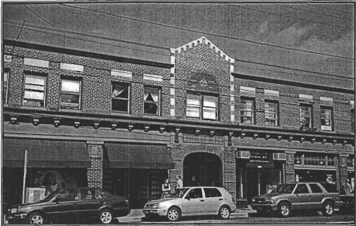
One of the many mixed commercial buildings along Hawthorne Boulevard that give Sunnyside its urban village character
