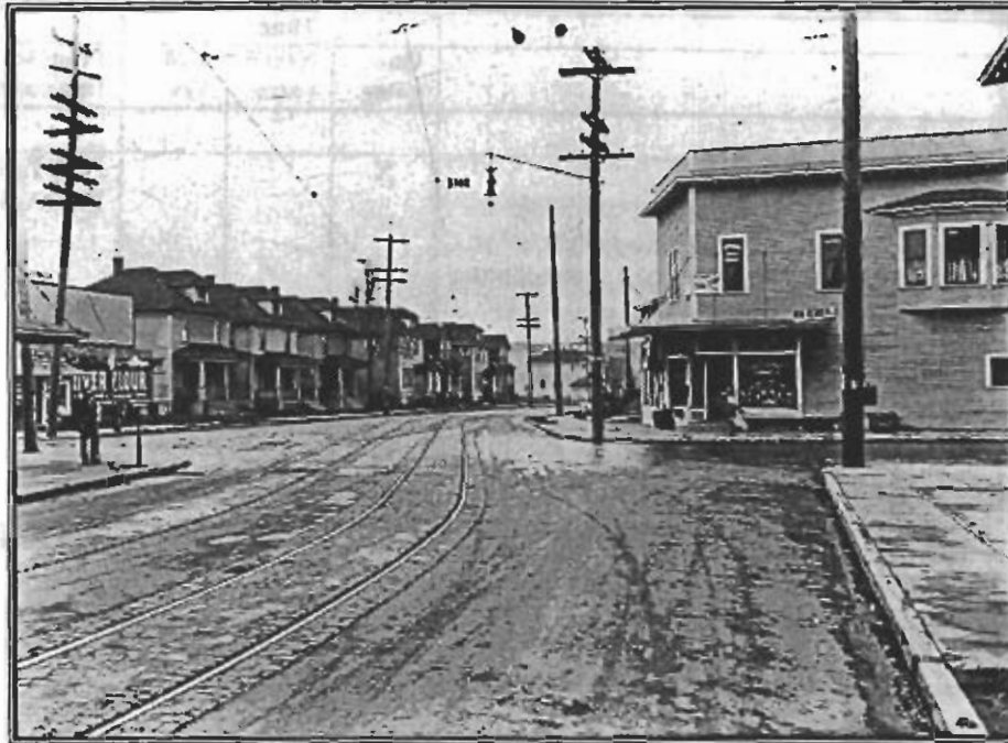
SE 39 th and Belmont, November 6, 1913, showing the alignment offset still existing today. Photo courtesy of Oregon Historical Society. COP 00029
