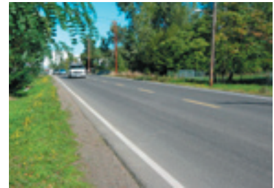
NE 47th Ave. does not have any sidewalks on either side.
