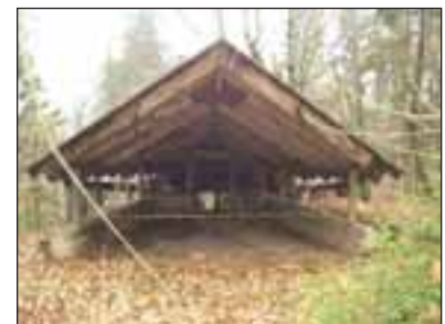
Schnabel Garage Structure
