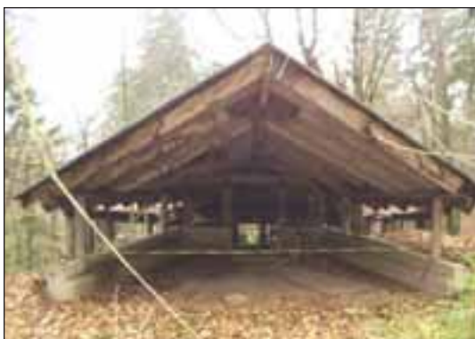
Schnabel Garage Structure
