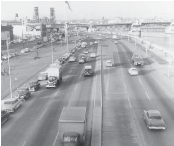
Top : The seawall under construction, 1929. Bottom : Six-lane Harbor Drive at the river's edge, 1958.
