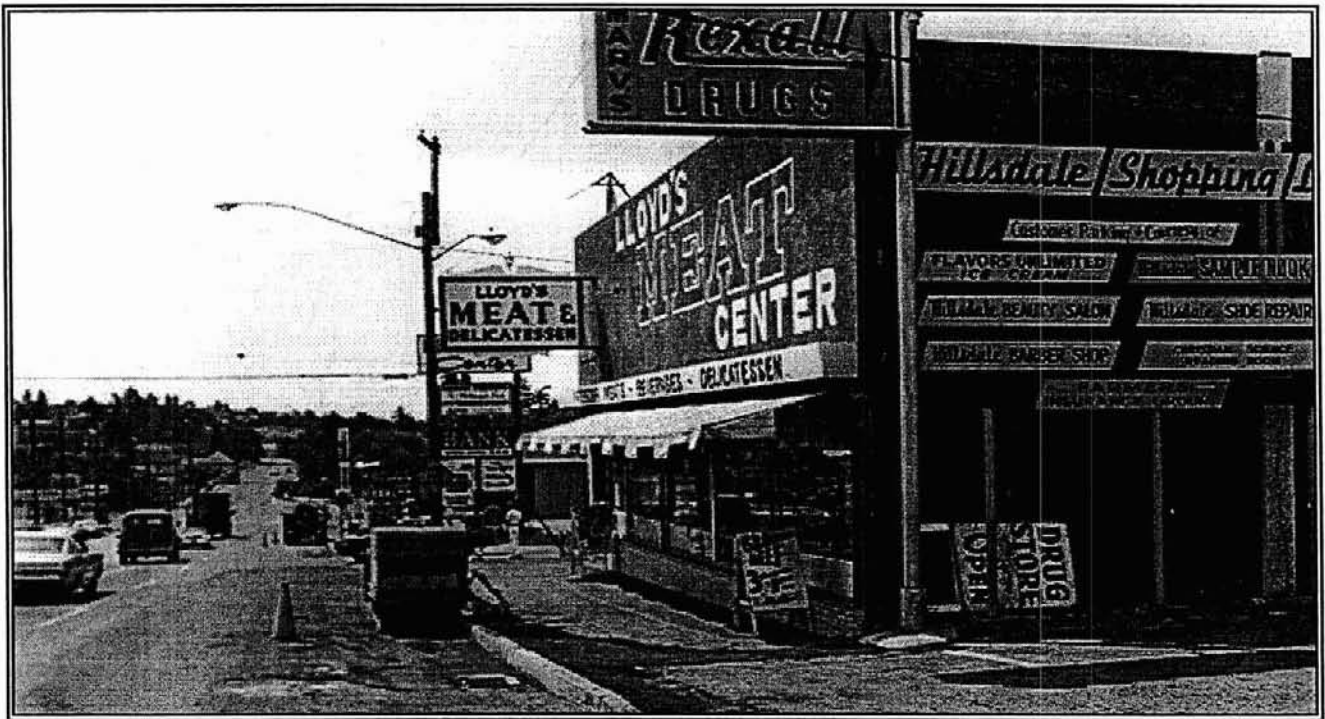
Hillsdale, 1968. Looking west on Capitol Highway towards the Bertha viaduct with Lloyd's Meat & Delicatessen in the foreground. Lloyd's was purchased in 1970 by the Edmunds family and turned into Poncho's Restaurant and Cantina. As of 1996 Joan Edmunds still operated Poncho's. Photo credit: City of Portland Archives & Records Center
