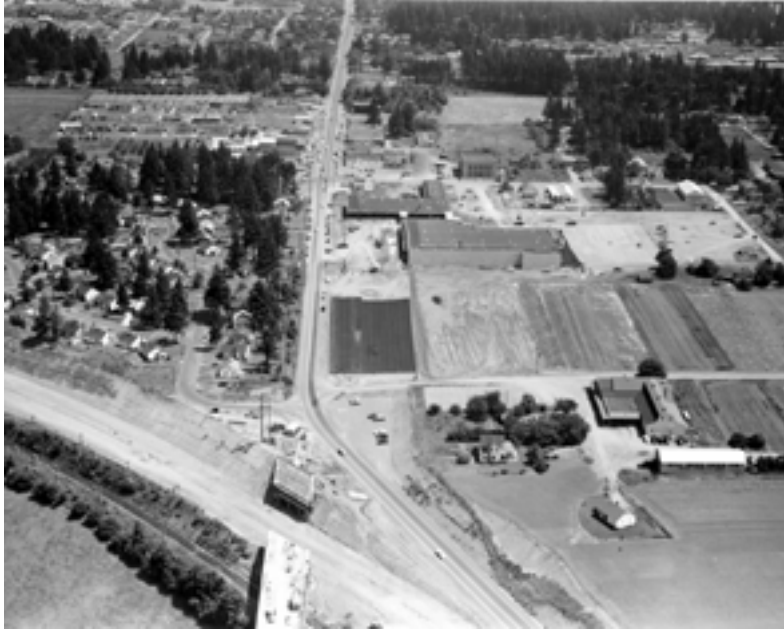
View east along NE Halsey. Both Fred Meyer, in the middle, and the I-84 Freeway, in the foreground, are under construction, probably the mid-1950s. Courtesy of Bob Earnest
