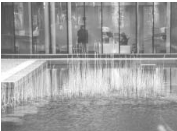
Stormwater retention pond incorporated into an office environment.
