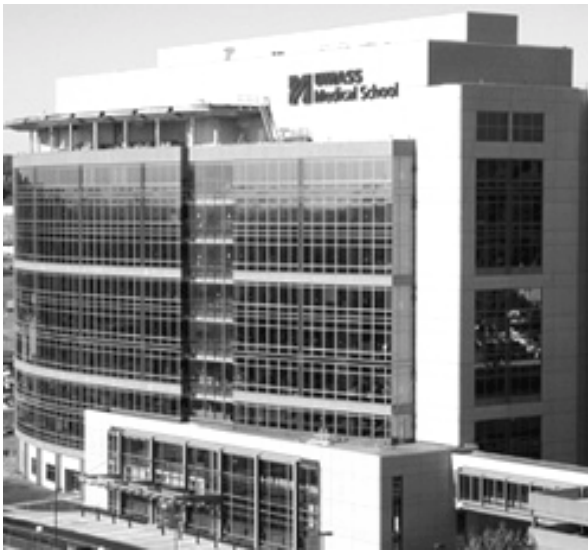
University of Massachusetts (Worcester) Research Laboratory Building
