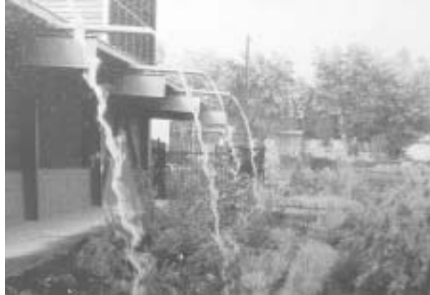
Vegetative filter and scupper, Bureau of Environmental Services Lab
