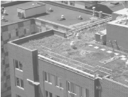
Eco-roof at Hamilton Apartments
