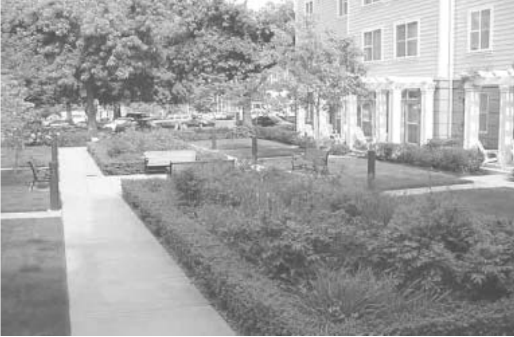
Landscaped stormwater detention facility at Buckman Terrace multi-family housing development.
