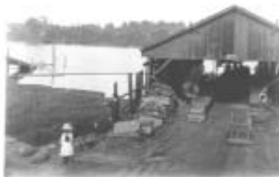
Power's Mill, early 20 th century
