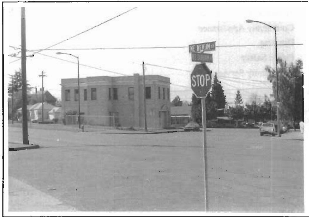
Neighborhood Focal Point at NE Dekum and NE Durham Streets (Photo by Paul Scarlett)
