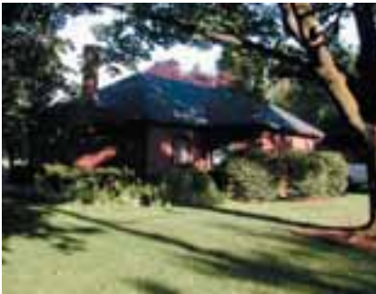
Maintenance Building, Summer 2002
