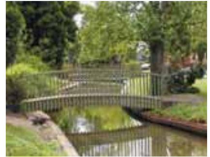
Crystal Springs Creek Crossing
