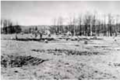
Casting Pond Construction, Ca. 1936
