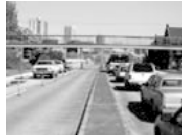
1. Naito Parkway looking north at SW Hooker pedestrian overcrossing.
