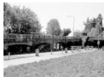
4. Foreground: Naito Parkway entering tunnel connection to southbound Barbur Blvd. Background: Naito Parkway northbound viaduct.
