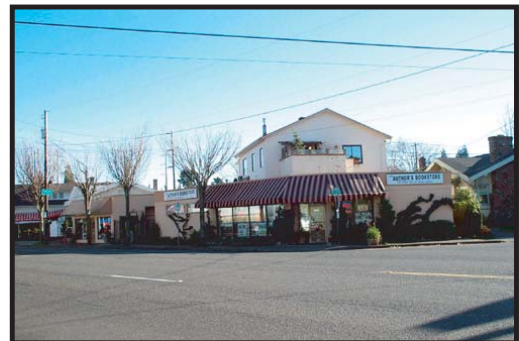
D Retail building on the south side of Sandy Boulevard.
