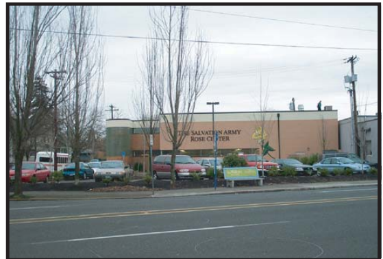
D View of Salvation Army on the south side of Sandy Boulevard.
