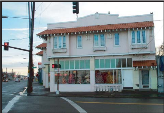
C Mixed-use building on the southeast corner.
