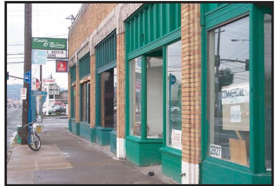
B View to the east of the north side walk
