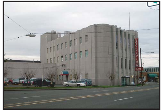
B The landmark Salvation Army Tabernacle on the north side of Sandy Boulevard.
