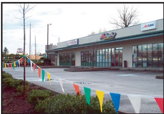
B Retail building on the south side of Sandy Boulevard.
