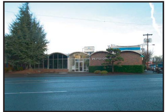
B View of Pepsi freight access on Oregon Street.
