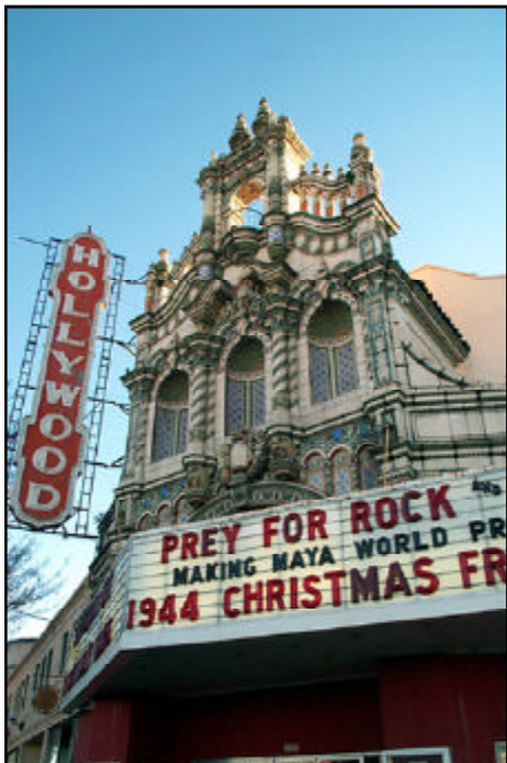
The Hollywood Theater is a corridor landmark.
