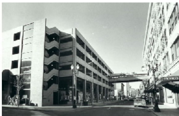
10th & Yamhill Garage and skybridge to the Galleria, 1984. Source: The Oregonian
