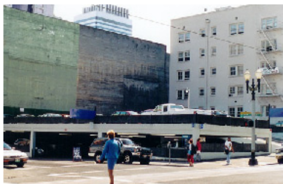
Parking garage at 938 SW Taylor, north and west sides, 2003
