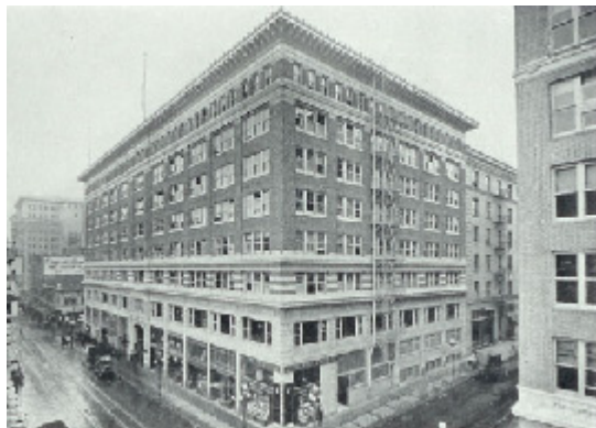
Morgan Building, west and north facades, 1914. Source: Nelson Photo Archive
