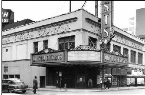
The United Artists Theater just prior to demolition, 1957. (The Oregonian)
