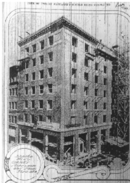
Hotel Willard (Morrison Park Building) under construction, ca. 1912. Source: The Oregonian
