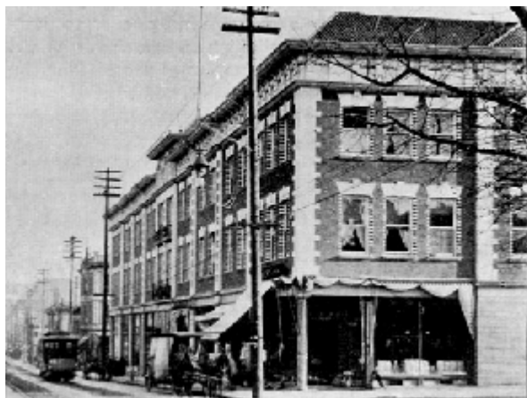
Selling-Hirsch Building, 1901. Source: Nelson Photo Archive
