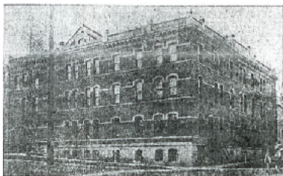
United Carriage Company Building, east and north facades, 1903. Source: Oregon Journal
