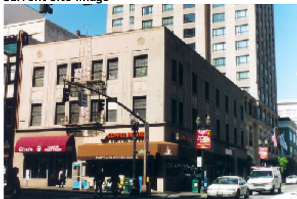
718 Alder Building, north and east facades, 2003
