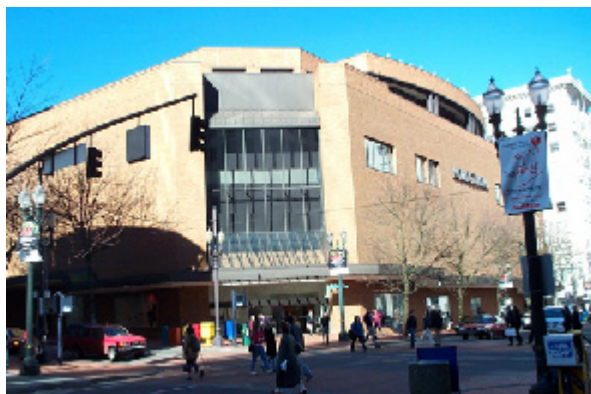
Nordstrom, east and south facades, 2004
