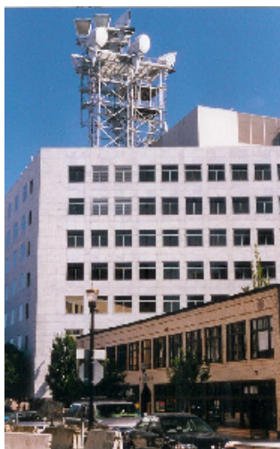
AT&T Building, south and west facades, 2002
