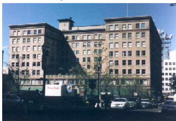
Pittock Block, south façade, ca. 2002
