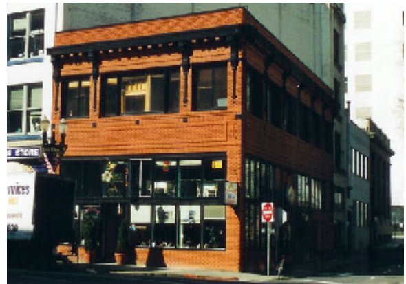
Blyth Building, south and west facades, 2003
