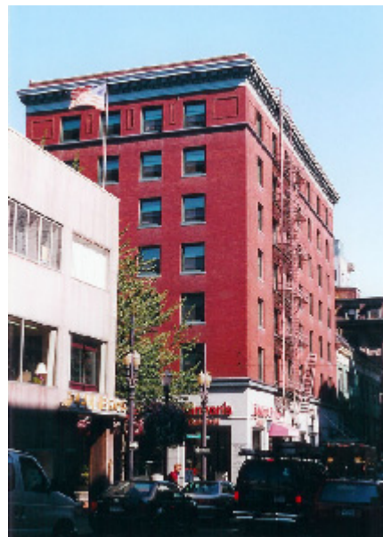
Morrison Park Building, east and south facades, 2002
