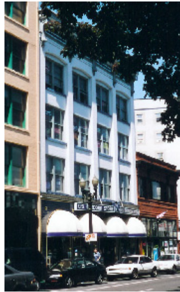
Fenton Building, east façade, 2003
