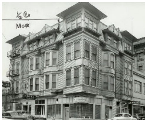
Beverly Hotel, just prior to demolition, 1954. Source: The Oregonian
