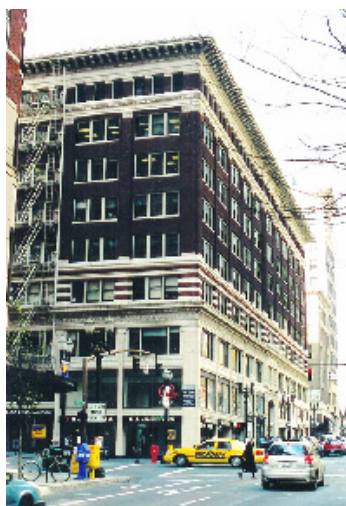
Morgan Building, east and north facades, 2003
