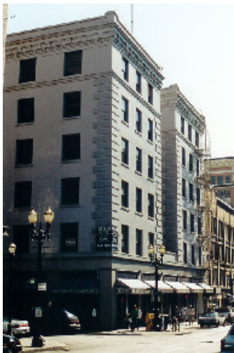
Medical Building (Park Building), south and west facades, 2003
