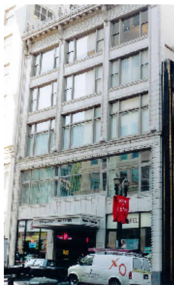
Liebes Building, east façade, 2003
