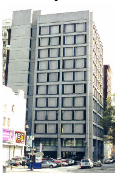
Qwest Building, west façade, 2003
