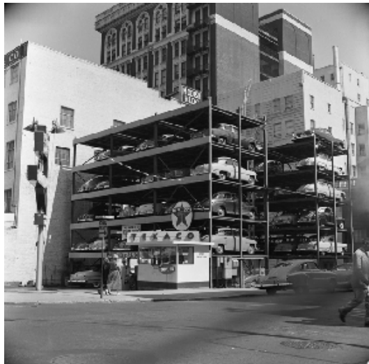
Pigeon hole parking structure, west and south facades, 1954. Source: Tom Robinson
