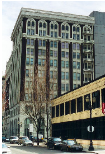
Capitol Building, north and west facades, 2003
