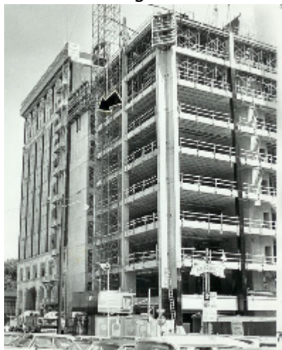
Capitol 2 Building, south and west facades under construction, 1969. Source: The Oregonian
