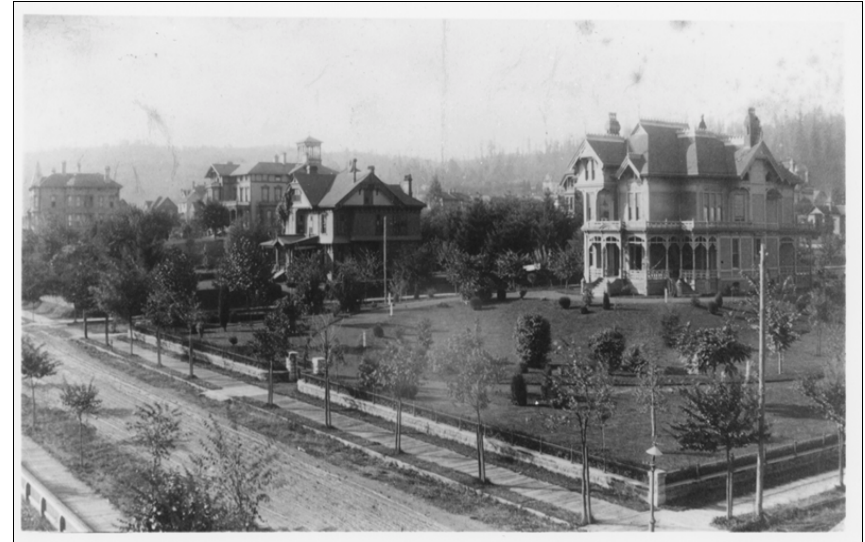
Looking southwest at NW 19 th Avenue from NW Johnson Street
