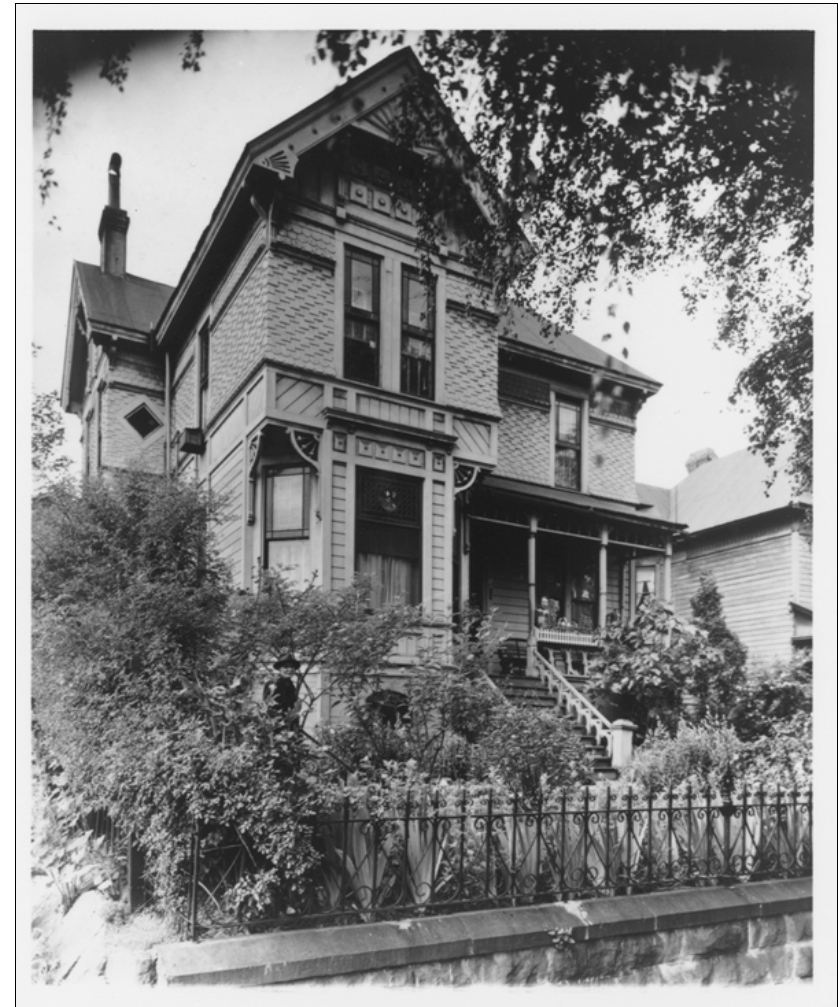
Looking westerly at 137 NW 20 th Avenue, no longer extant
