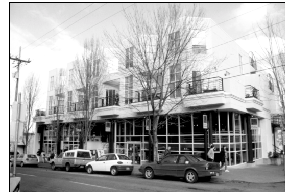
L & G Ltd. Partnership Building, 404-410 NW 23 rd Avenue
