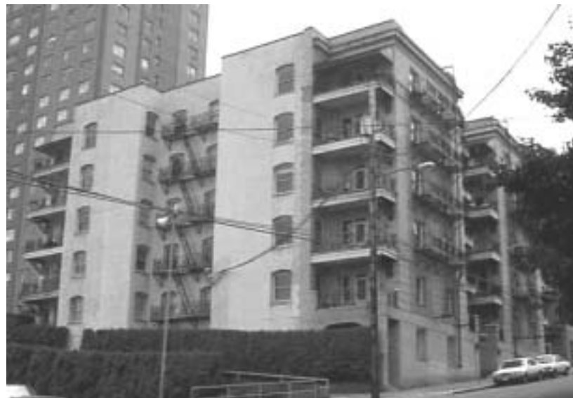
The Fordham Apartments at 742 SW Vista Avenue are located at the northwest edge of the district, which is defined by historic multi-dwelling development.
