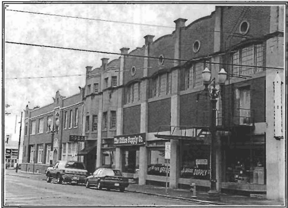
Simple bold structural expression in the design of those buildings used for industry helps to blend them with commercial buildings in the District.
