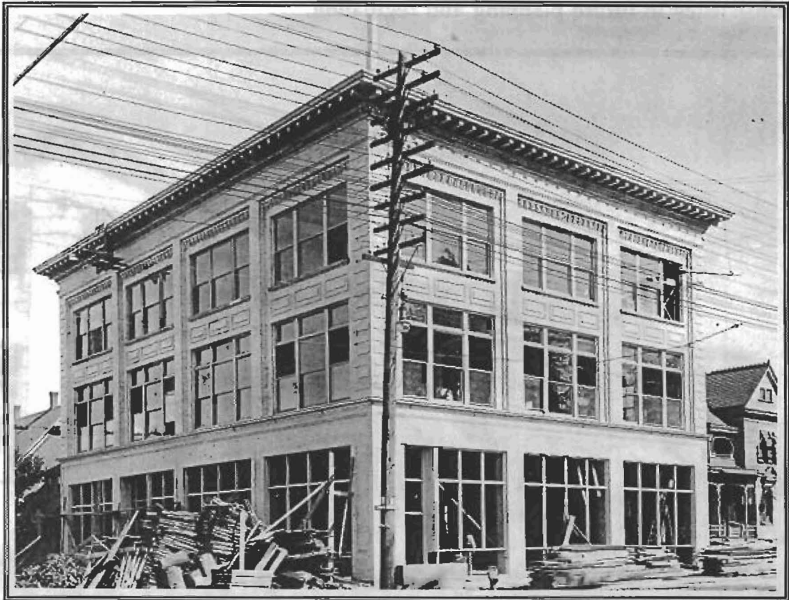
U.S. Laundry Building under construction in East Portland. The Building, located at Yamhill Street and Grand Avenue, is a good example of care in design and the choice of materials resulting in a handsome work of architecture. (OrHi 009234)
