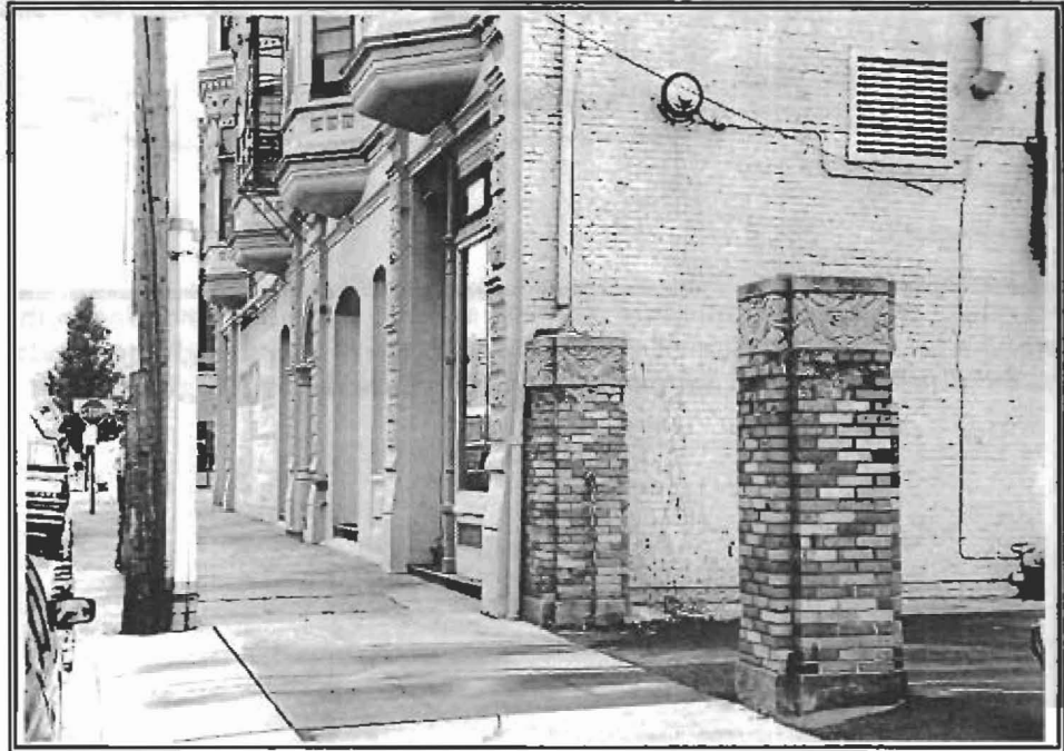
Remnants of a building once located on this site are retained to create a gateway to a parking area.
