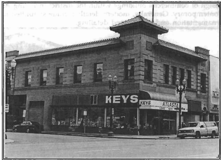
Attractive turn of the century commercial building with recent awning addition illustrates how an inappropriate awning design may detract from a building's architecture.
