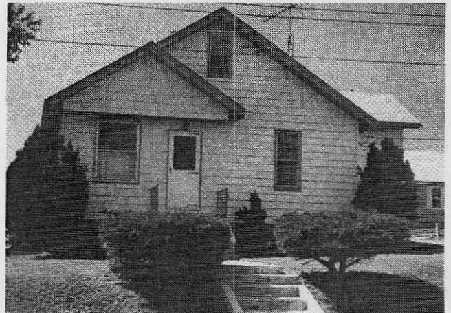
VARIANT 4. Inappropriate siding and covering trim boards, porch changed, windows removed, brackets removed, colonial storm door, wrought iron railing.
