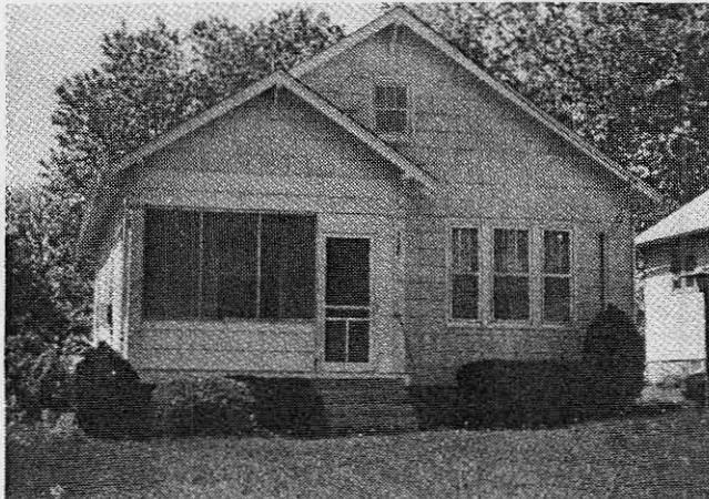
VARIANT 1. Inappropriate siding and enclosed porch.
