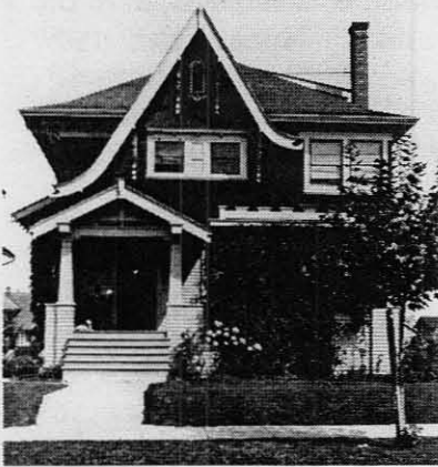
Holcomb House, 1990 SE Mulberry Avenue, c. 1915, Oregon Historical Society, ORHI 63002
