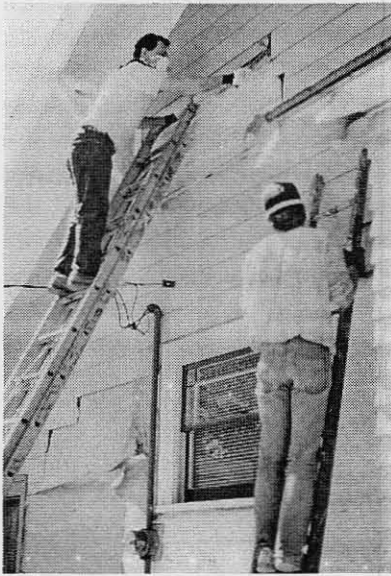
Ladd neighbors assist in removing asbestos siding, an annual Historic Preservation Week project.
