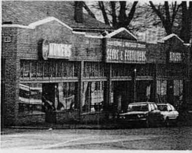
Typical streetcar era commercial building with vintage signs.
