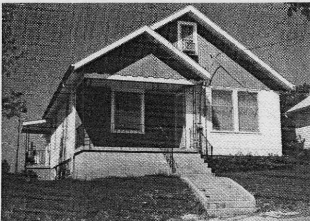
VARIANT 3. Inappropriate siding with vertical boards in gables, air conditioner, windows replaced, brackets removed.
