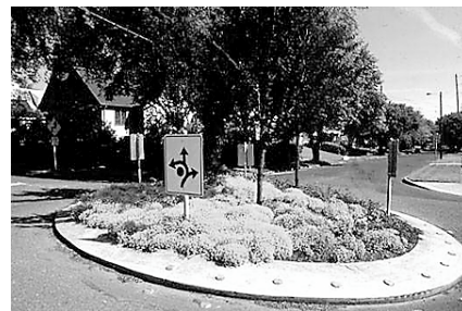
Traffic circle at NE 37 th and Wisteria
