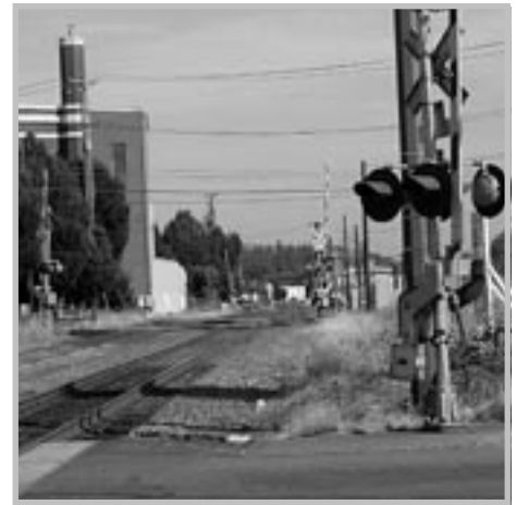
At-grade railroad crossing in SE Portland.
