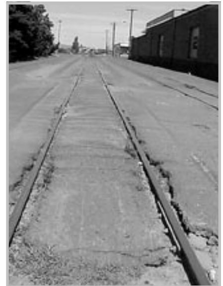
Deteriorating pavement on N. Bradford.
