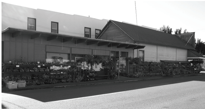
The Bookmine's addition does not take away from the original false front structure that sits on the first half of the lot and demonstrates what an appropriate addition within the district should look like. The addition is simple, low in profile, and completely hidden from Main Street.
