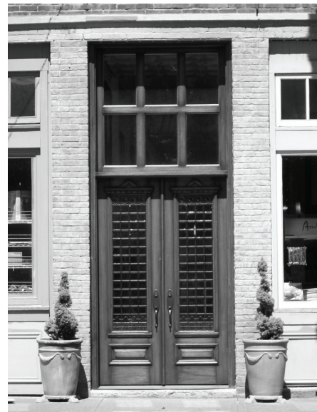
The doors replaced on the Old Town Club Building are great examples of era appropriate pieces. The doors are too fancy for downtown and the historic hotel that was originally at this location; however, the addition of these doors and the reopening of the transoms brought the façade of the building back to the most historically significant time period for this structure.
