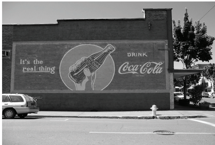
Brick that was not historically painted should remain bare, however, any historically painted brick, like the above Coca-Cola sign, should be preserved.
