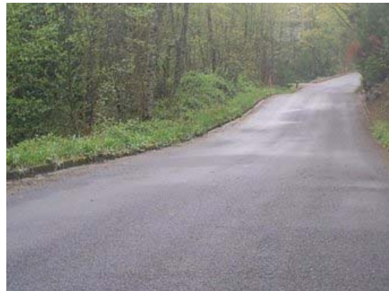
Soil creep: undulating pavement and curbs
