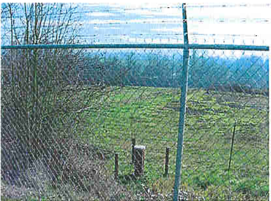
Methane vents on landfill site
