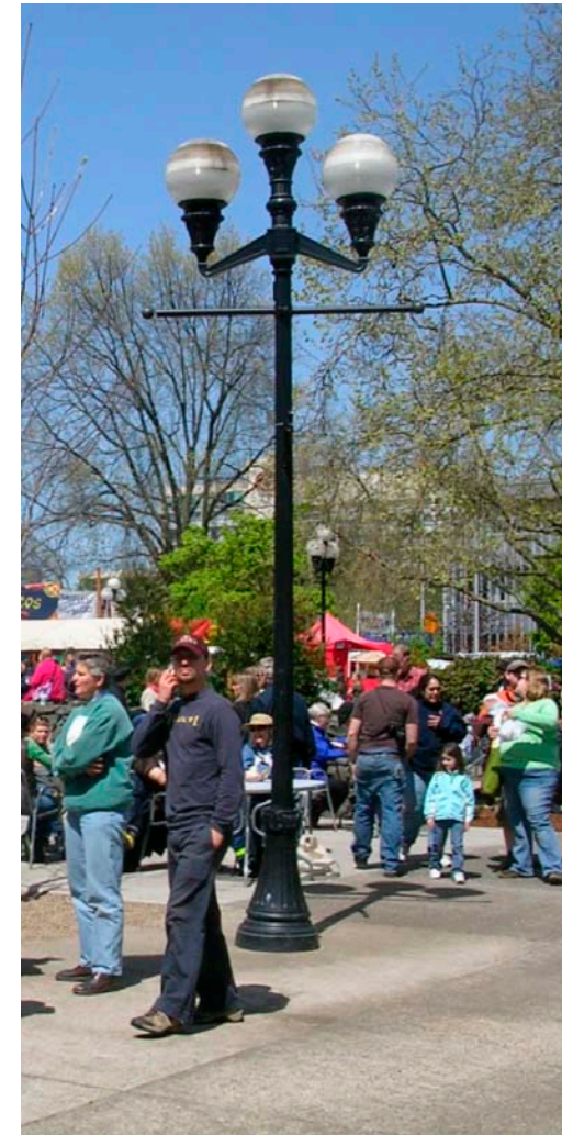
Typical existing street lamp
