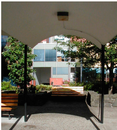
Existing shelter lighting
