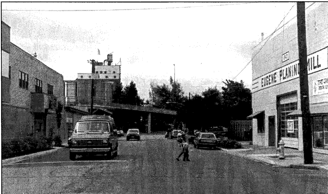
The Eugene Planing Mill established in 1906 grew to occupy about a four block area. The area now contains a diverse mix of uses.
