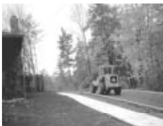
A separated sidewalk was one element of this Local Improvement District in Southwest Portland.
