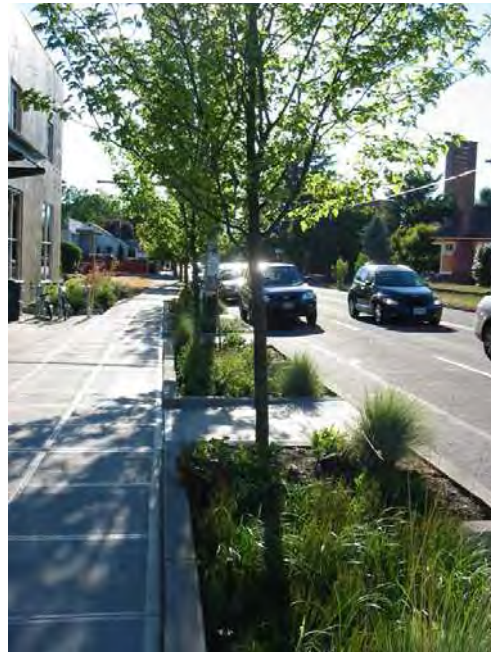
Landscaped planters within the planting strip manage stormwater and serve as a visual amenity
