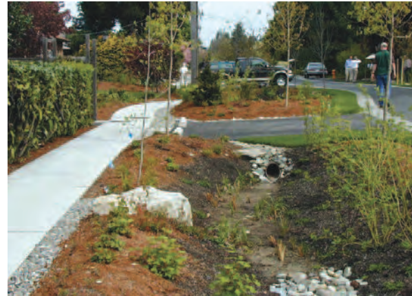
Curbless green streets allow water to flow freely into vegetated bioswales, where it is allowed to seep into the ground or pass beneath driveways into other swales
