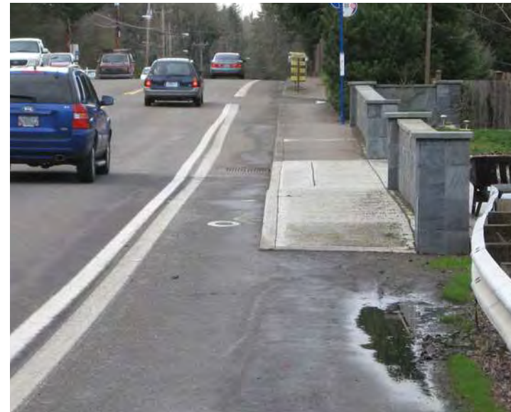
Obstructions in the bike lane and poor transitions make cycling difficult
