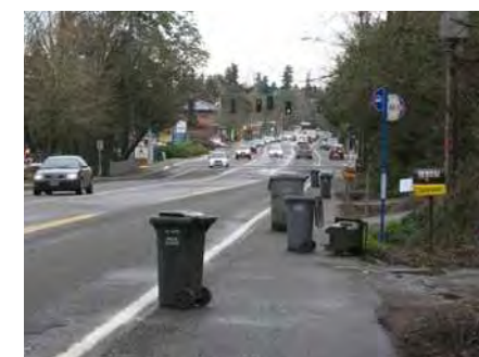
Obstructions in the bike lane make cycling difficult
