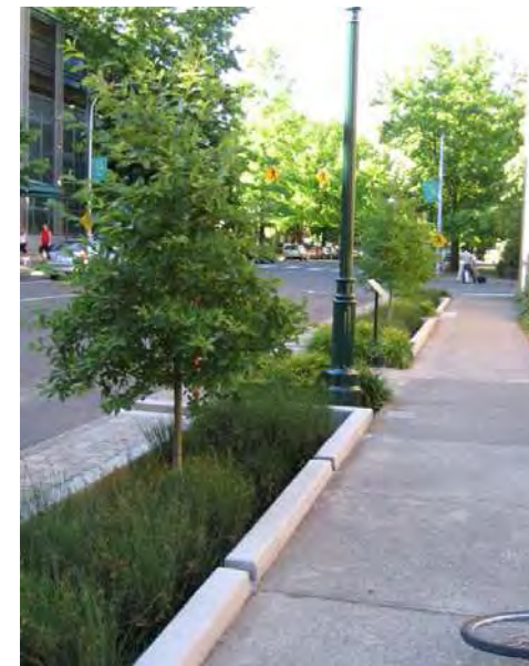
Stormwater planters are often linked together, so that when one planter fills up, water flows down into the next planter
