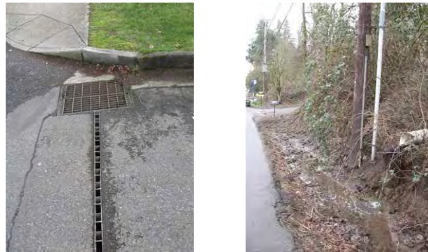
Stormwater is currently directed into traditional sewer systems or drainage ditches; instituting green / sustainable stormwater management practices can help protect the various waterways that cross beneath OR 43 in West Linn
