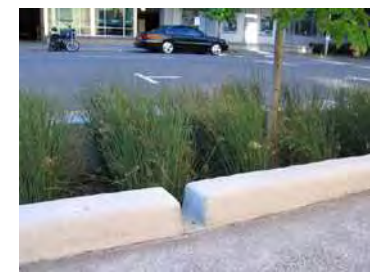
A slotted curb adjacent to the sidewalk allows the planter to collect runoff from sidewalks as well as street runoff
