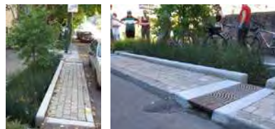
A curb cut channels street runoff into structured planters, where it is allowed to percolate into the soil
