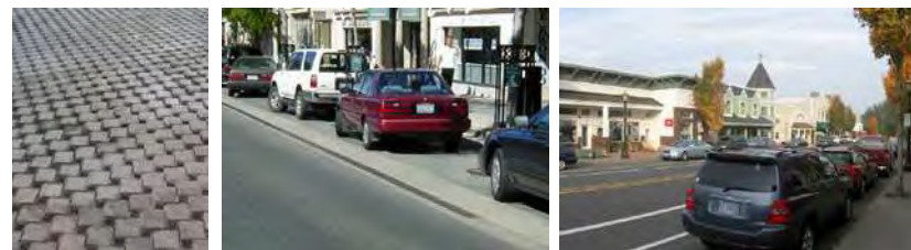
Permeable pavers can be used in parking areas to mitigate stormwater runoff
