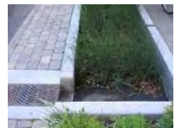
A curb cut channels street runoff into structured planters, where it is allowed to percolate into the soil
