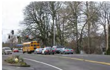
This curb/median prevents left turning movements to/from this shopping center driveway; shoppers instead must use the left turn lane and signal at the Hidden Springs intersection
