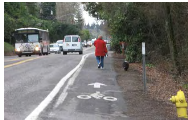
Existing sidewalk conditons along OR 43
