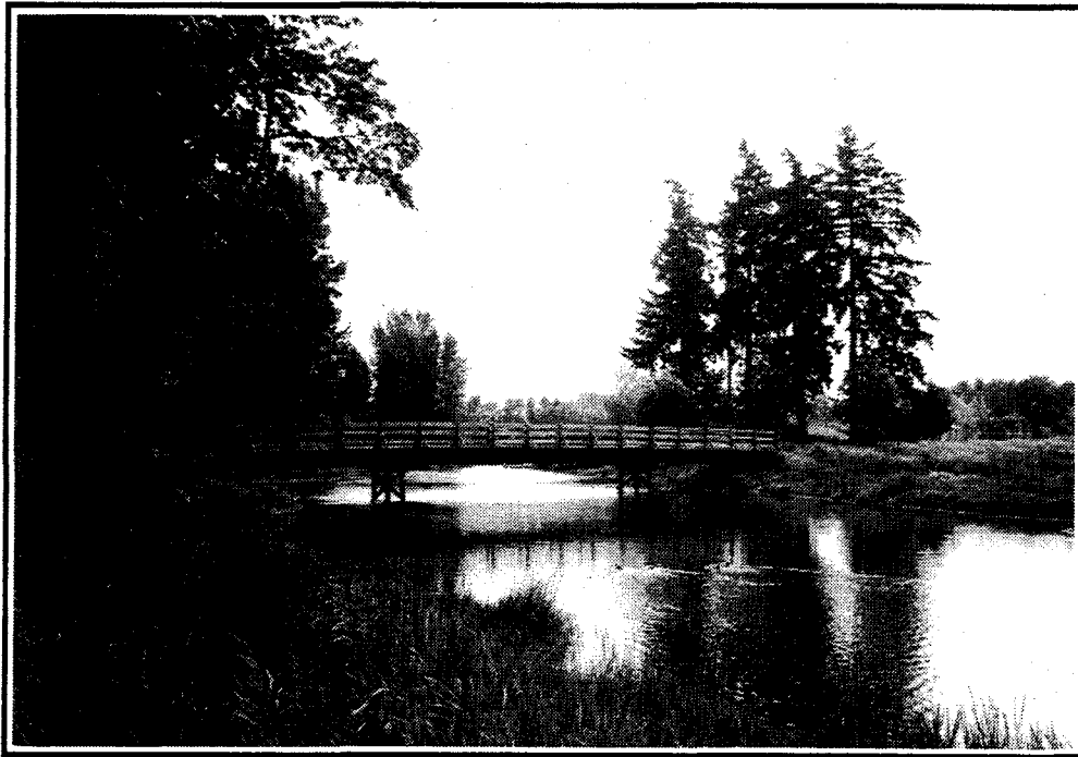
Pedestrian bridge over canoe canal in Alton Baker Park.
