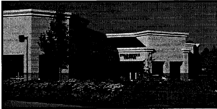
EXISTING "TANASBOURNE TOWN CENTER" EAST OF NW 185TH
