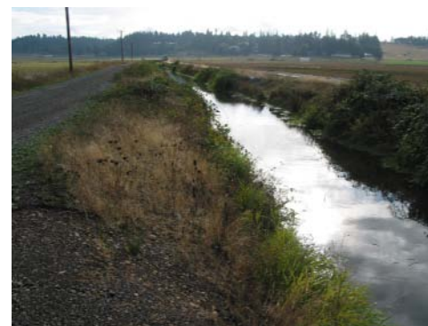
Figure 8. East/West Ditch (Ditch 6)
