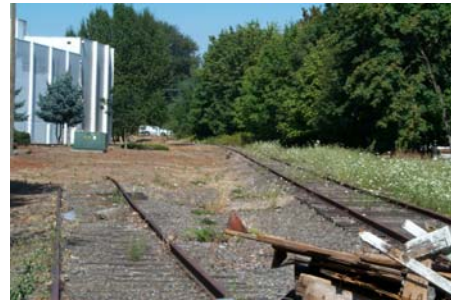
Abandoned Railroad Right-of-Way West Salem Gateway Area
