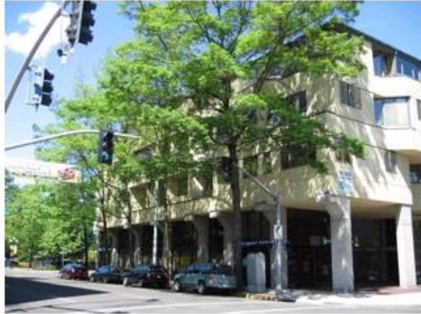
Parkview Office Building 101 E. Broadway, Eugene
