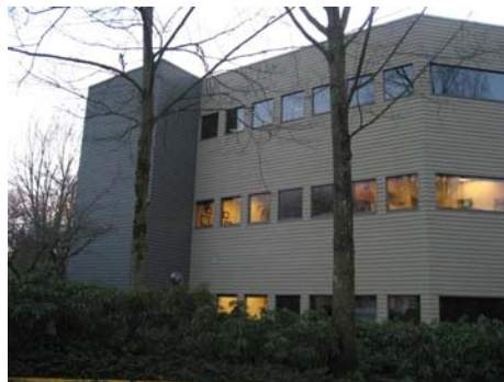
Figure 5: Northbank Office Building, 44 Club Road, Eugene
