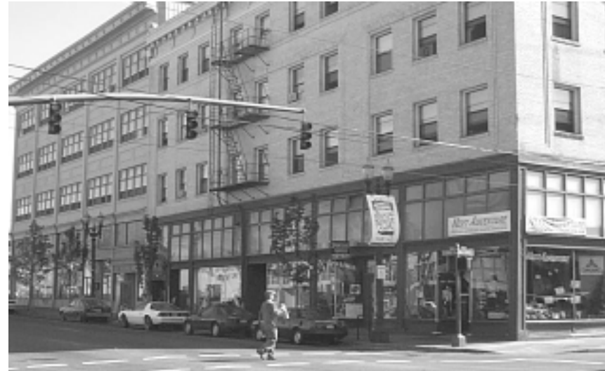
Differentiated sidewalk-levels along SE Grand and SE Stark Avenues
