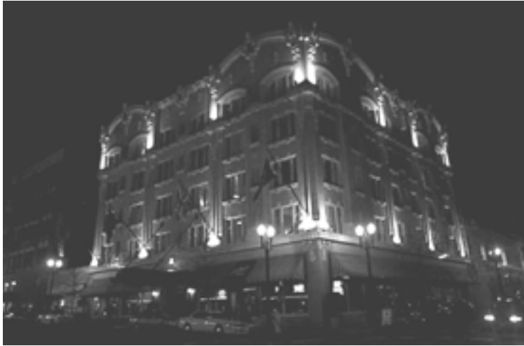
The Governor Hotel in downtown Portland uses a series of "uplights" to emphasize the vertical components of the building's structure at night.
