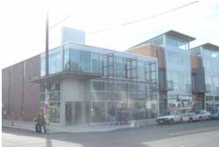
The Hawthorne Condominiums building at SE 34 th and Hawthorne has incorporated a two-story retail space at the building's corner at 35 th Avenue. This space offers a large, highly visible location for special tenants to capitalize on the area's high levels of pedestrian and retail activity.
