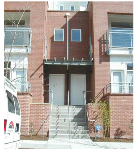
Not Recommended: Colorless and unarticulated entry doors do not convey a welcoming appearance (NW Northrup and 23rd, Portland)
