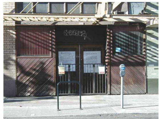
Not Recommended: Fixed security bars on windows and storefronts and security gates in front of the entrances (N Denver and Kilpatrick and NW Couch and 4th, Portland)
