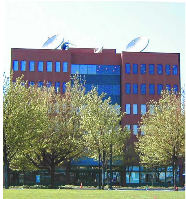
Not Recommended: Rooftop equipment visible and not integrated into building design (SW 2nd and Stark, Portland)
