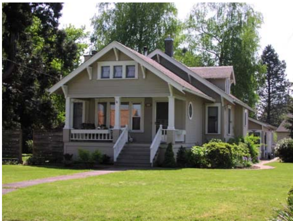
Charles T. Hall Residence - 1918
