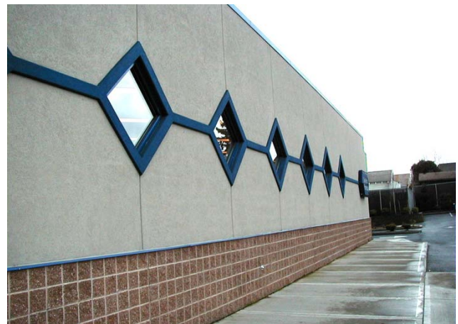
Not Recommended: Horizontal wall character exaggerated by the lack of wall definition and the oddly sized and shaped windows (N Lombard and N Denver, Portland)
