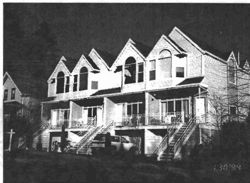
Townhouses with partially excavated parking help to retain neighborhood scale and maintain the human connection to the street.
