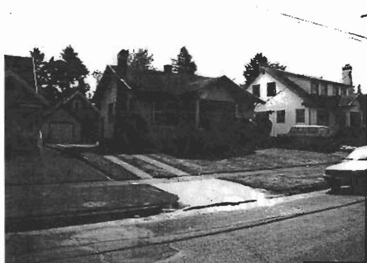
Tire tread drives, rather than a fully-paved driveway, minimize interruption of the streetscape & decrease run-off.
