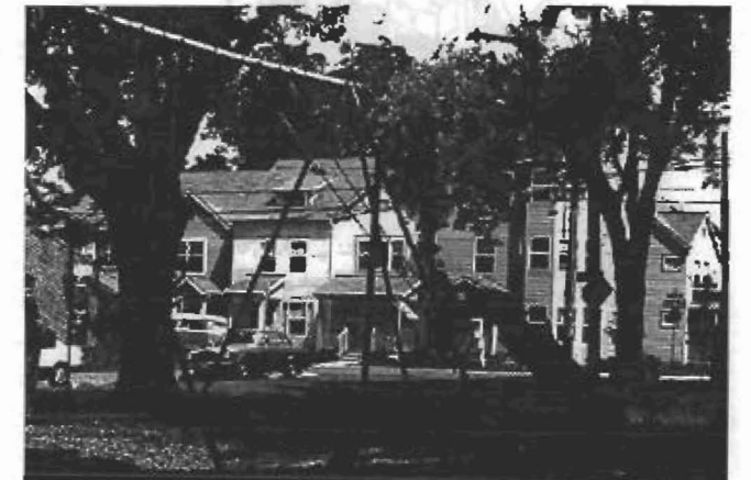
Family-sized units next to park with a playground.
