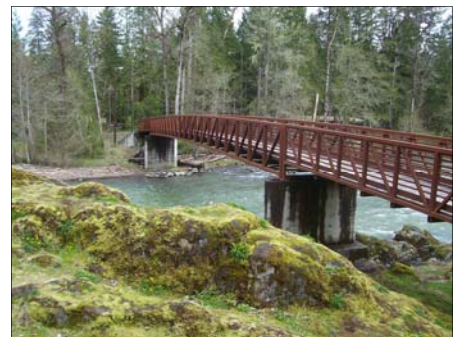
Jim Tharp Memorial Footbridge at Greenwaters Park. Photo: R. Ojerio
