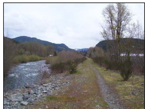
Salmon Creek South Levee. Photo: R. Ojerio
