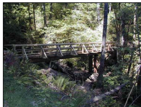
Bridge on the North Fork Trail. Photo: Middle Fork Trail Crew.
