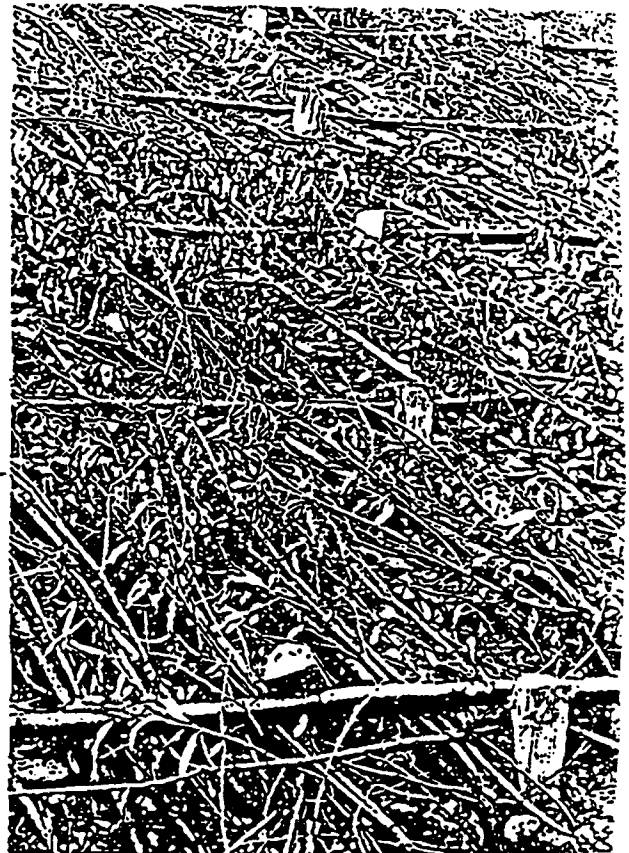
137 Detail of a newly constructed brushmattress.
