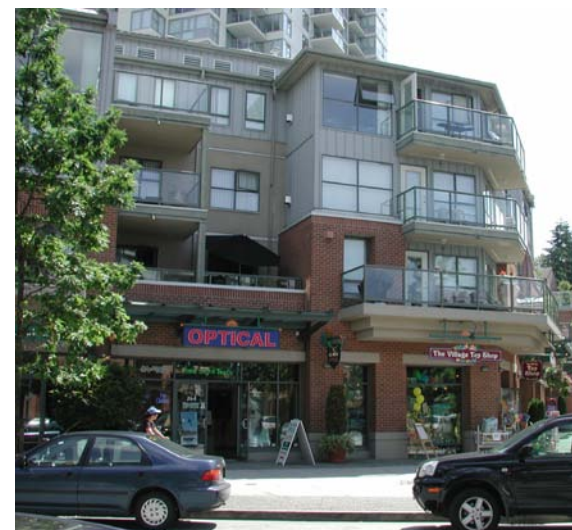
Mixed-use urban development in the Canadian city of Port Moody, British Columbia.
