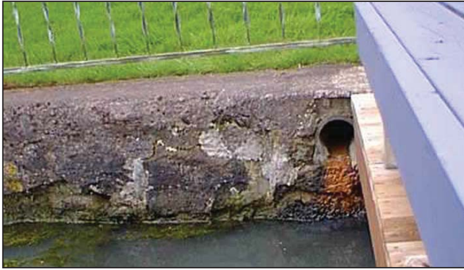
Oswego Lake Outfall Improvements Main Lake
