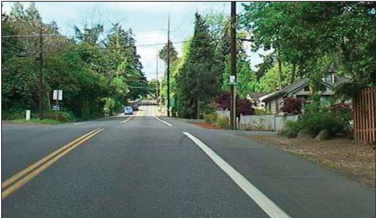
McVey Avenue at Lake Front Road (Unfunded)
