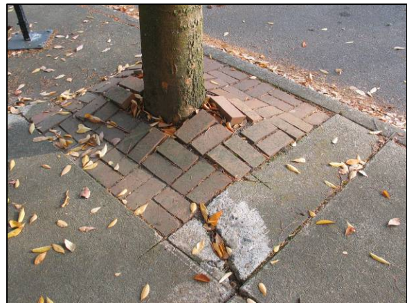
Sidewalk uplift on B Avenue.
