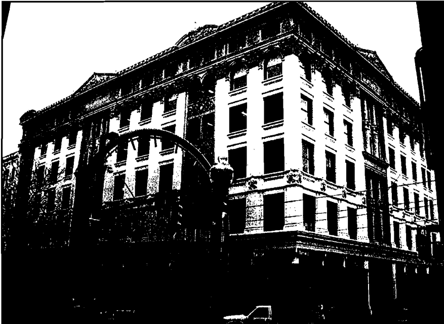
Illustration 5-29 "Faddish" Public Art and Loft Buildings with Integrity in the Market Center Historic District, Flathman, 2007
