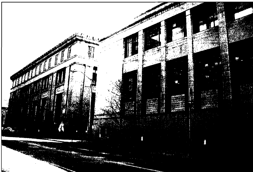
Illustration 3-34 Annex Exterior, Flathman, 2007
