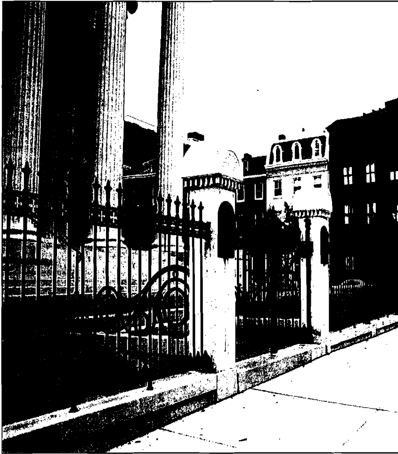
Illustration 5-31 Gates Discourage Use of the Basilica's Terraces, Flathman 2007
