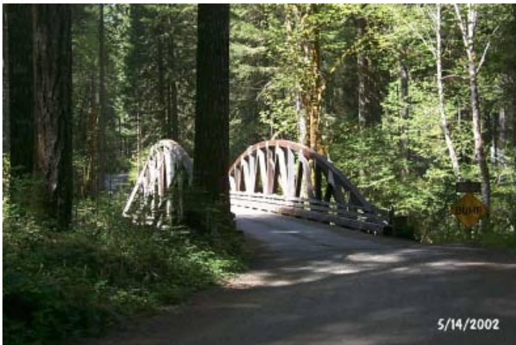
View from Delta Rd. looking south.
